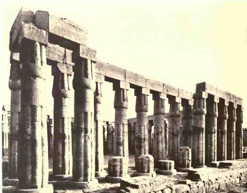
The Colonnade of Amenhotep III at Karnak Temple, with its massive papyrus columns.
