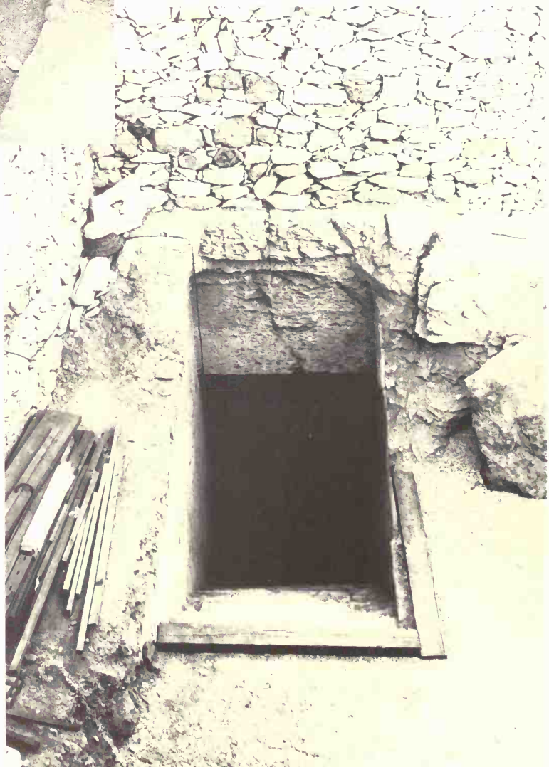
The stone of the tower had been of a soft kind, and the masonry was of a bad quality. The well opening was of a bad quality, and the stone lining was of a bad quality. The wooden frame was of a bad quality, and the well-poles were of a bad quality.
